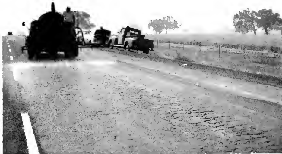
Watering the pavement
